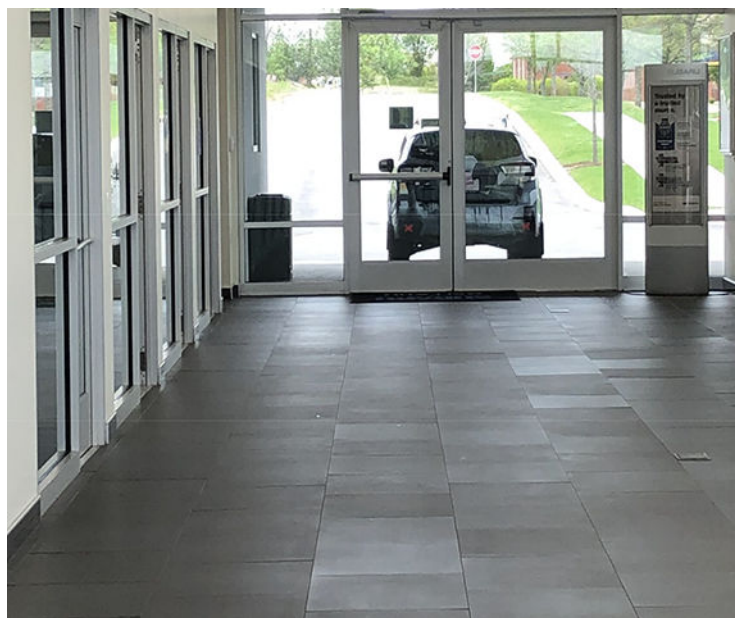
FIG. 1 Low Angle Light Defect Visible in an Installation
